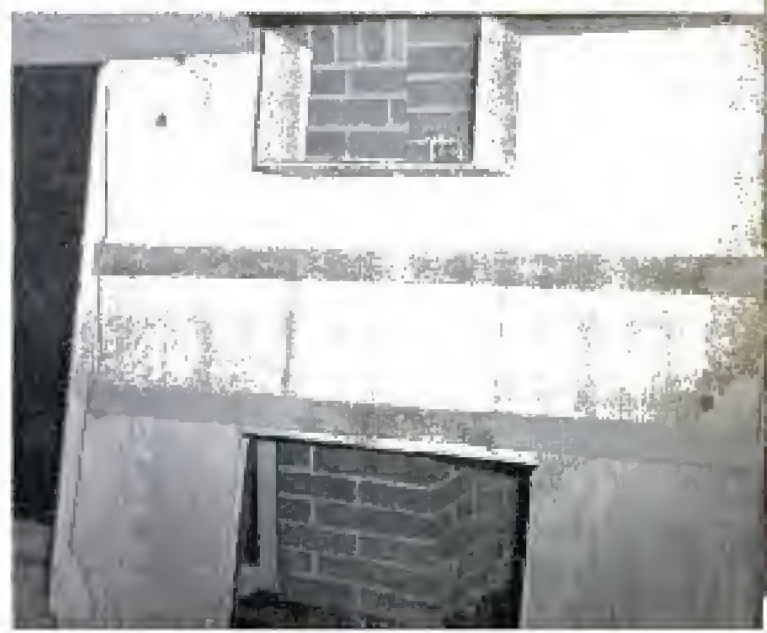
A back view of the front panel of the fireplace shows how panels are braced with 1 x 3 lumber
